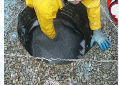
SPI goes the extra mile. These Petro-Barriers™ were custom installed at a depth of 6'. Reinforced grating was bolted into the pipe and the Petro-Barrier™ media installed. This resolved an issue with the perforated pipe that was already installed.
