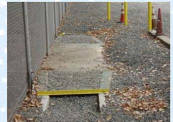
A Drainage trench 12" deep runs around the south side of this substation for water drainage. The trench leads to (2) 30" wide x 5' long storm water drains. Grating is installed in the drains and crushed stone is used to fill the trench to slow water flow. The Petro-Barrier™ media is installed and topped off with clean crushed stone. This system has been exposed to flooding since its installation with no drainage problem.
