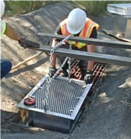
Lowering the StormWater **Petro-Barrier™** into the Drain Housing.
