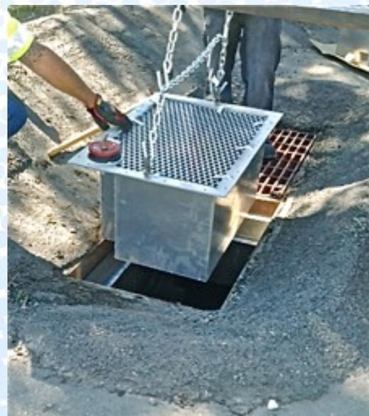
Lowering the Storm Water **Petro-Barrier™** into the drain housing.
