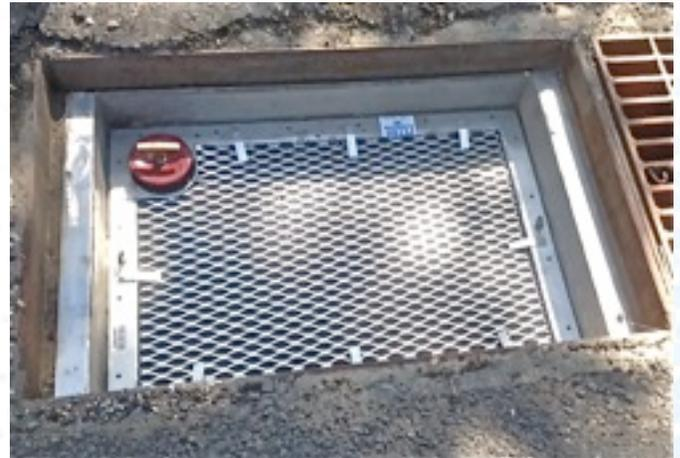
StormWater **Petro-Barrier™** Properly Fitted with Emergency Bypass Valve.
